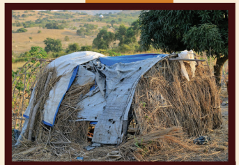
Leaky old hut
