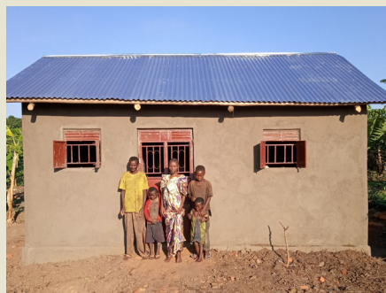
Old and New Shelter
